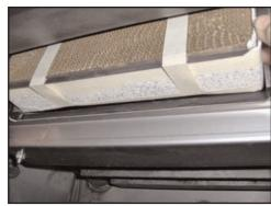
Since the combustor is only 2" deep, there is ample room to lift the new combustor into place. REMEMBER TO HAVE THE TAB ACROSS THE BOTTOM EDGE OF THE COMBUSTOR AS IT IS INSTALLED. Slowly push the combustor in at the top, apply even pressure to the left and right corners. This will allow for a better view of the bottom edge for the final fitting. DO NOT FORCE THE COMBUSTOR INTO THE DOME. TAKE YOUR TIME AND WORK IT INTO PLACE SLOWLY.
